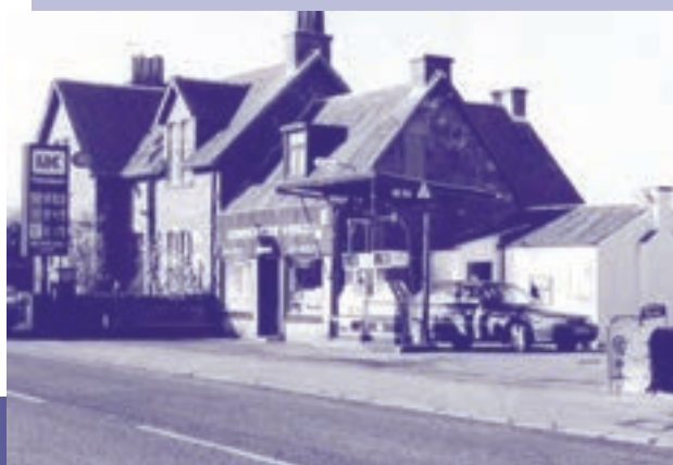
Lomond View Stores and Petrol Station, Main Road, Gartocharn
